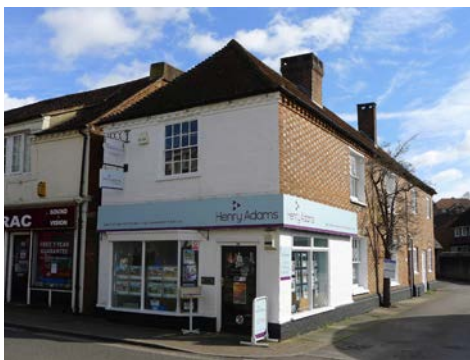
This building's orientation, brick eaves cogging and flared brick headers are all characteristic details.
